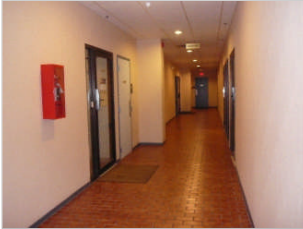
2nd Floor Corridor
